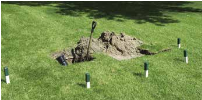
Mark off repair areas.
